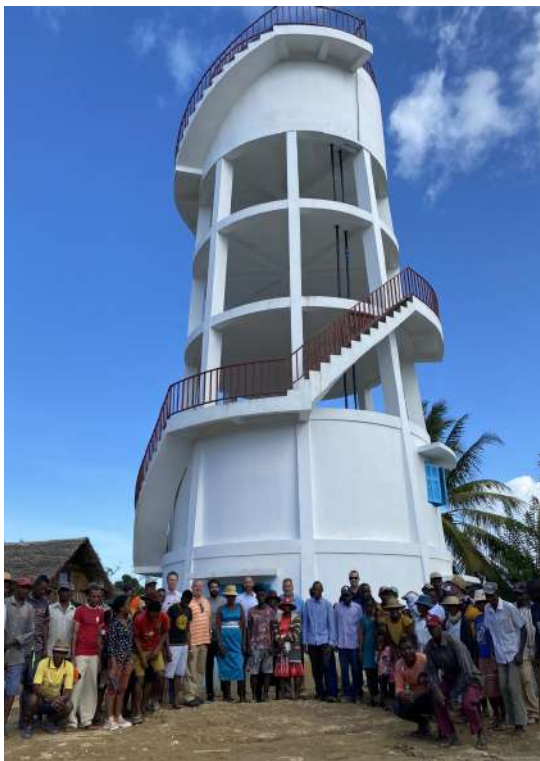
Newly completed solar-powered clean water system in the village of Ampohibe, Madagascar
